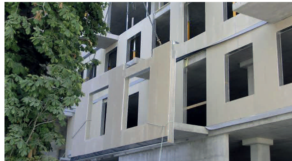
A residential building in the City of Kharkiv
