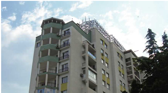
A residential building in the village Nikita
