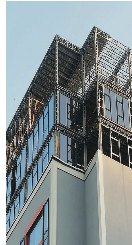
A superstructure of 3 floors in the City of Kamianske
